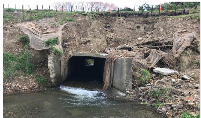
Figure 2 - Scour to Back Road and damage to the Culvert
