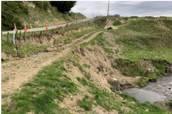
Figure 2 - Scour to Back Road and damage to the Culvert
