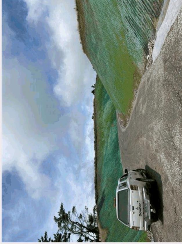
Grass starting to grow and stabilise batters after one week
