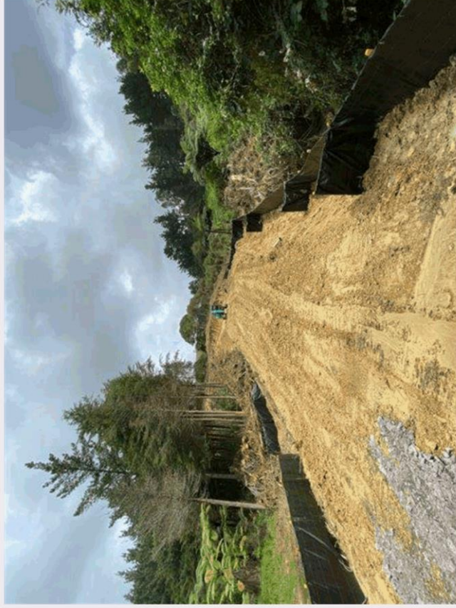
Super silt fences installed around access track construction to control any sediment runoff
