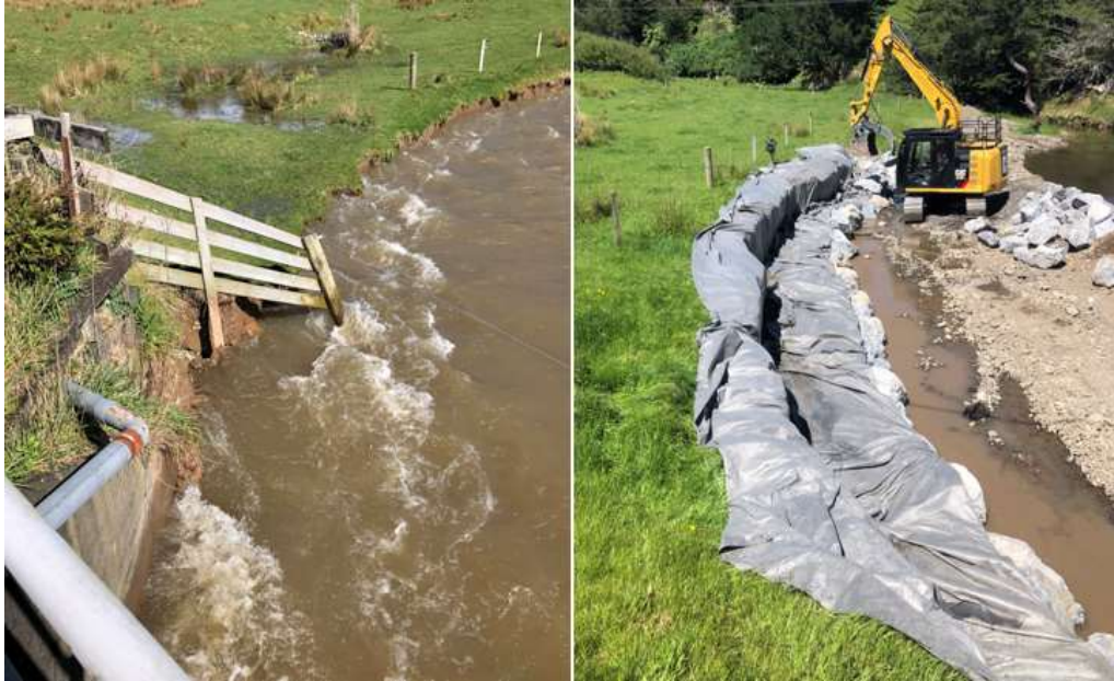
Figure 4: Turitea Bridge #2 embankment repairs
