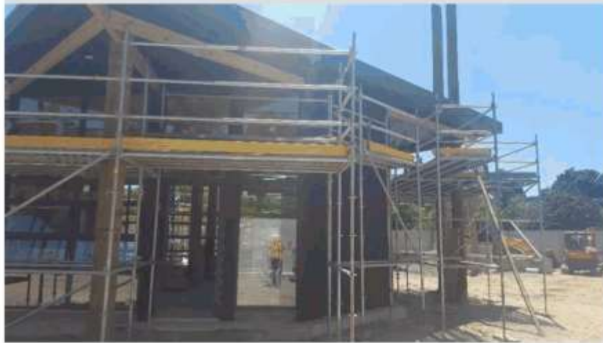
Exterior large windows have been installed along with glazing – 23/11/2017
