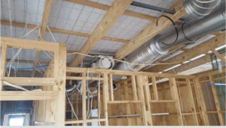
All in-wall services has been installed before plasterboard – 09/11/2017
