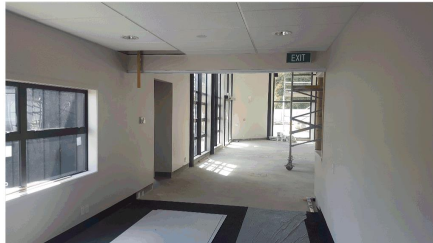
Operable doors to be installed, suspended ceiling installed – 15/02/2018
