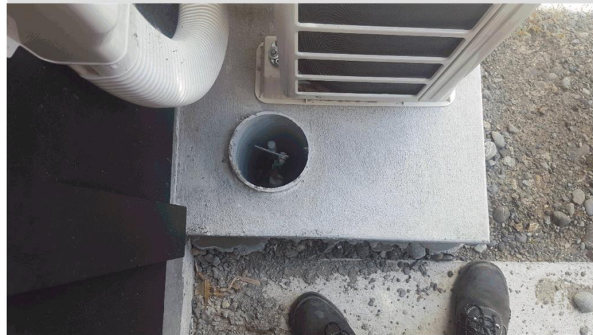
Outdoor HVAC units installed and grounded – 15/02/2018
