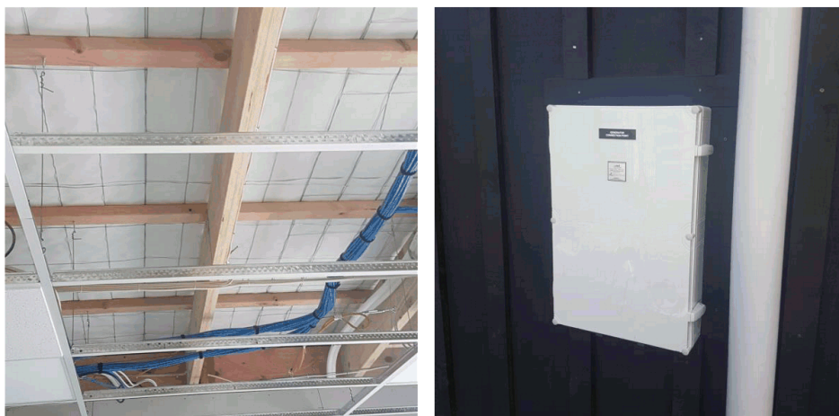
Figure 6 Underlying roof purlins (left) and the main switchboard/point of connection for the PV system on the external wall on the Northwest corner of the building (right)
