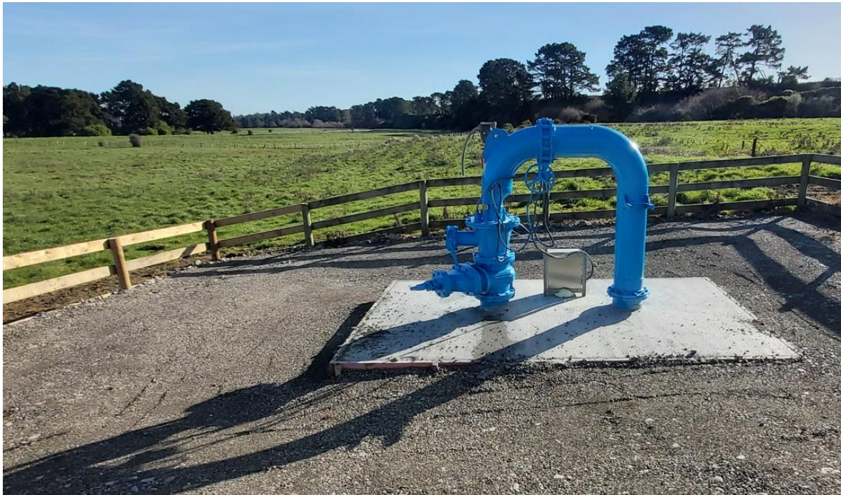
Figure 2: Ashhurst Bore post upgrades to achieve compliance (e.g. fence, concrete plinth, sealed casing)
