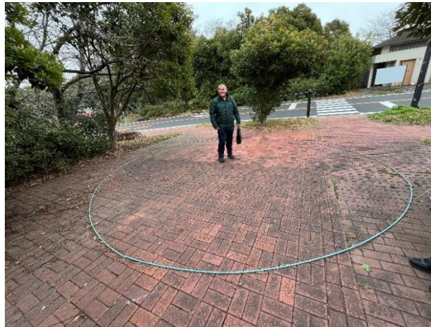
Figure 33- The rope circle depicts the size of the incoming sewer pipe; the bricks are made from the ash by-product from the Biosolids incineration.
