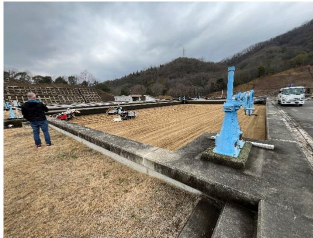
Figure 30 - Labour intensive slow sand filters at Nishino WTP
