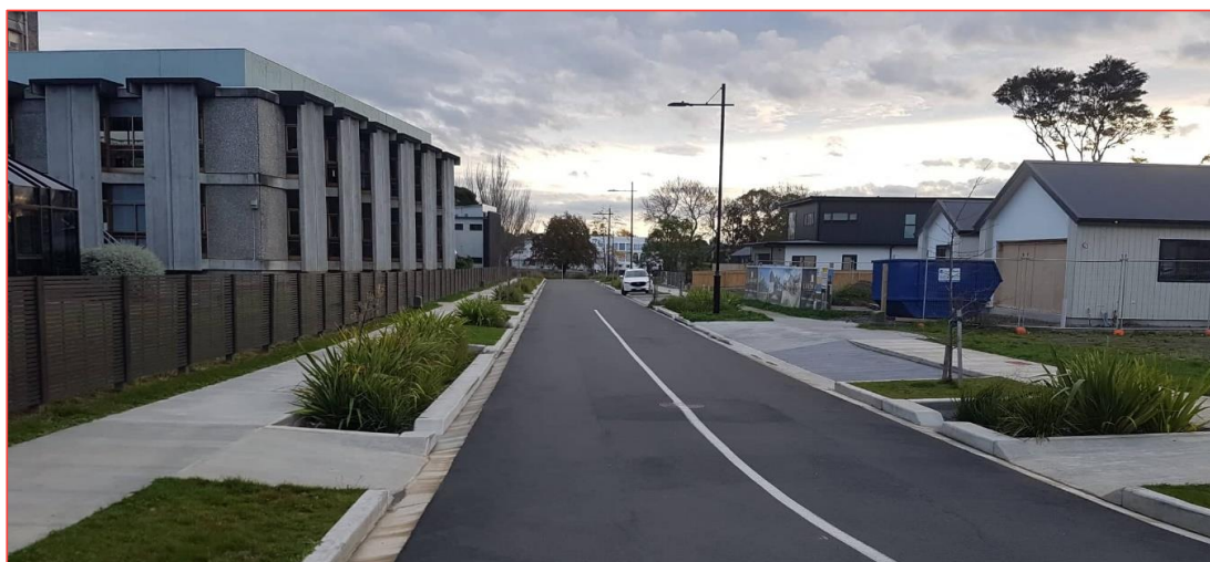
Figure 4-8: Example of a 13m Roading Corridor - Hokowhitu Lagoon Development
