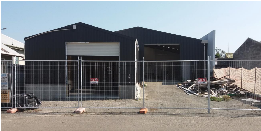
Photograph 13a: 3-5 Roxburgh Crescent – Asbestos cement sheeting on exterior of a building on site identified in Property files held by PNCC
