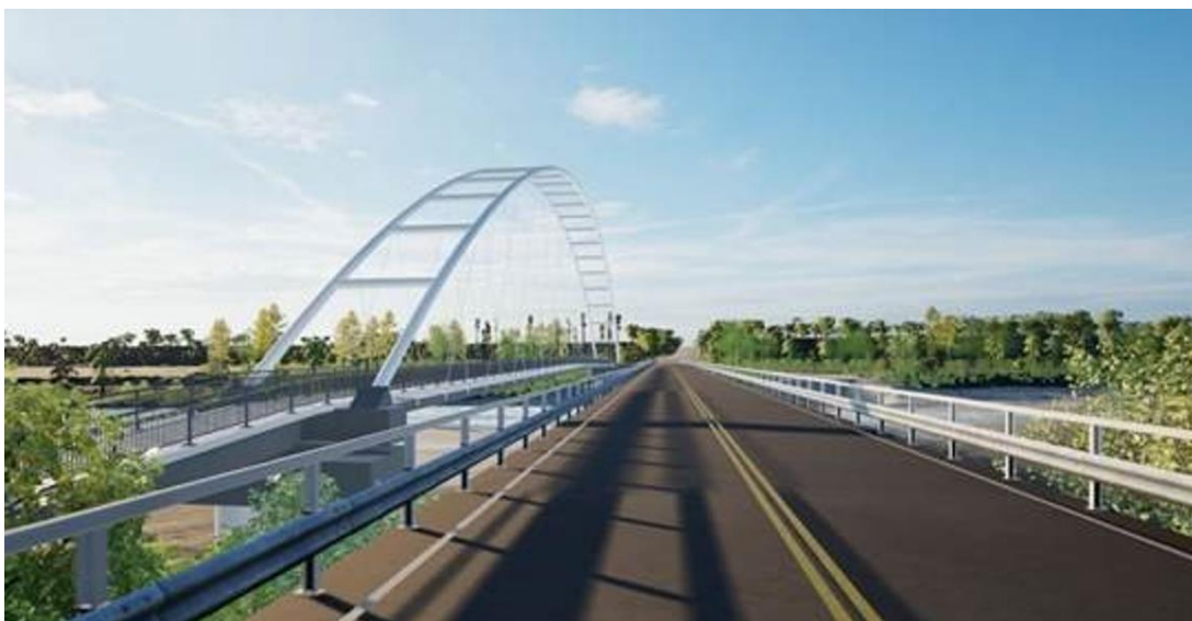
Figure 2: Pedestrian/Cycle Bridge at Ashhurst
