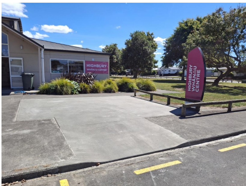
New pram crossing to access HWC and sports fields. In past users had to mount the kerb or go out to the road to access a pram crossing
