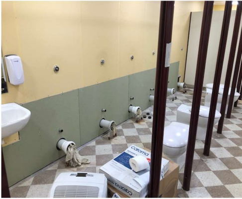
New Toilet Pans being installed
