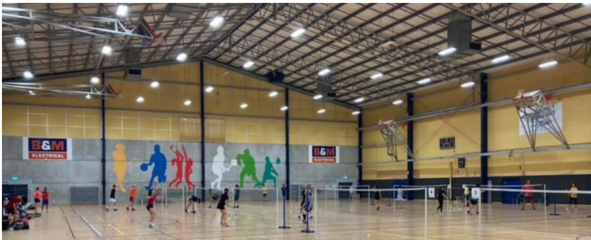
Figure 5: Portal Frame Structure Example - Arena 4 B&M Centre
