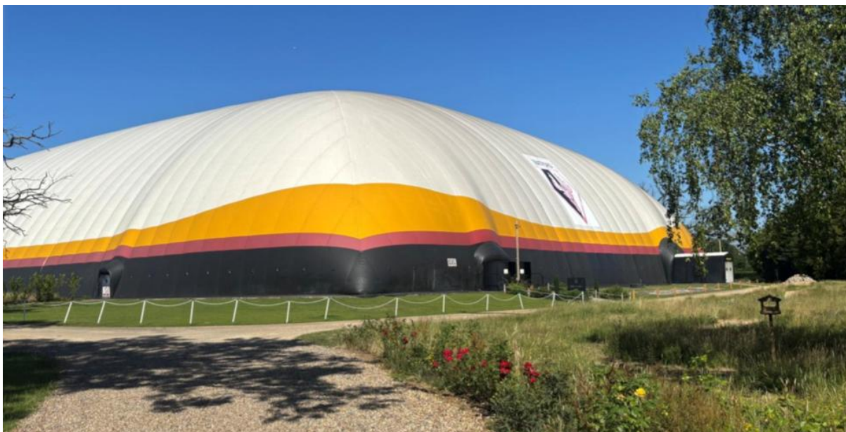
Figure 3: Air-Supported Structure Example (Exterior) – Watford Football Club, London
