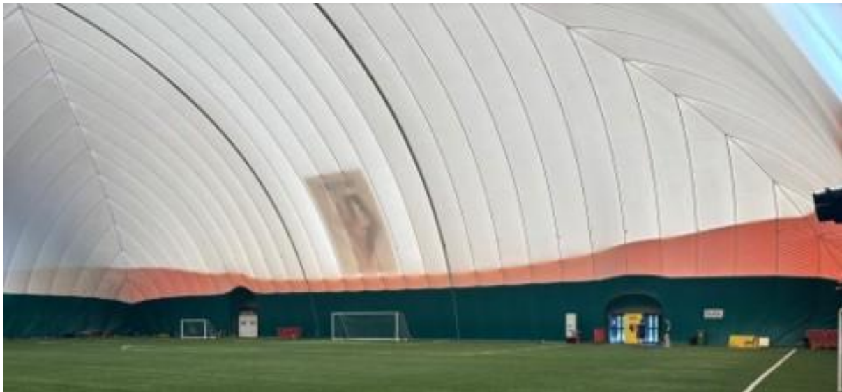
Figure 4: Air-Supported Structure Example (Interior) - Watford Football Club, London
