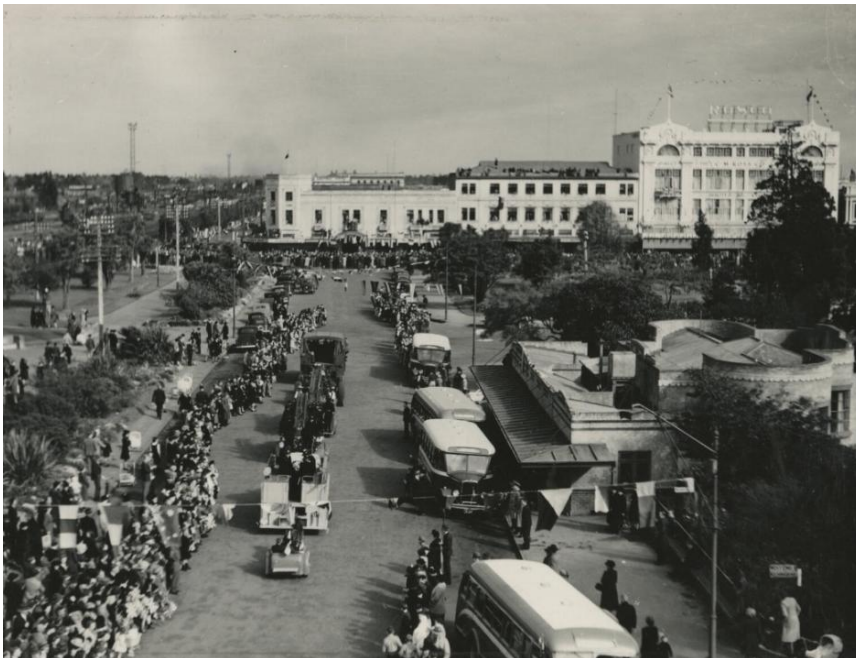
Figure 9 The facilities were no doubt well-used on 9 May 1945, as the procession around The Square to celebrate peace with Germany in World War Two passed by. The bus shelter at the rear of the Ladies' Rest is also visible in this image.
