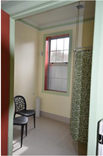
Figure 22 The accessible shower room in the former attendant’s office. Anna Renton-Green, 25 September 2025, HNZPT.
