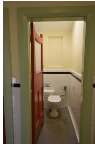
Figure 21 A typical toilet stall; note curved tiles between wall and floor. Anna Renton-Green, 25 September 2025, HNZPT.
