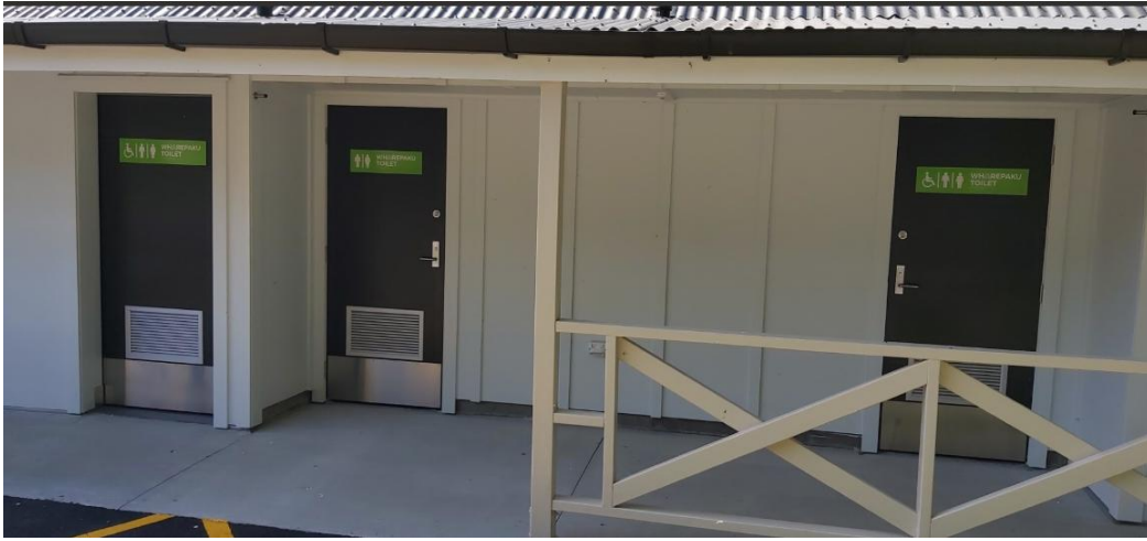
Example of the kick back plates installed at Kelvin Grove Cemetery
