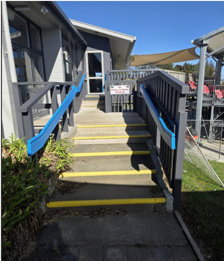
Access Improvements carried out at Colquhoun Park
